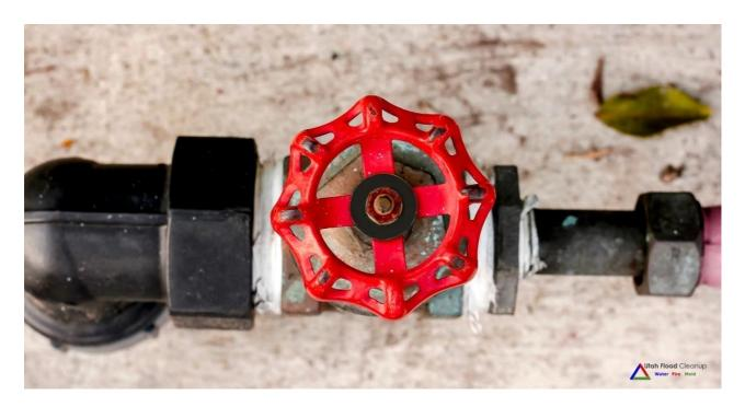
There are multiple water shut-off valves in your home. Together, these regulate the water flow rate through plumbing pipes, faucets, and water outlets going into appliances throughout your house. The shut-off valves enable you to cut off the water going to a particular faucet or other water outlets. This is a critically important capability in a <u>house flooding</u> emergency when a repair or replacement is needed, and during periods when your house will be vacant for an extended period.
