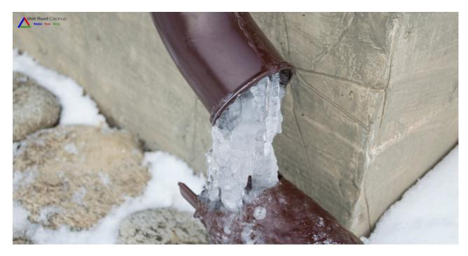
If temperatures drop to freezing or below, water pipes can freeze, expand, and burst, causing <u>flooding from a broken pipe in your home</u> when the frozen pipe begins to thaw. It can create a huge cleanup problem, damage or destroy furniture and other personal property, undermine the support structure of the home, and cause mold to spread throughout the affected area of the home. Here's information on how to thaw a frozen pipe before it causes major water damage.
